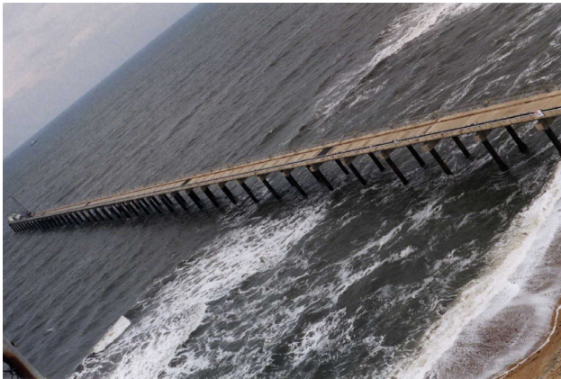
Figure 4. The Duck FRF pier seen from a nearby tower.
