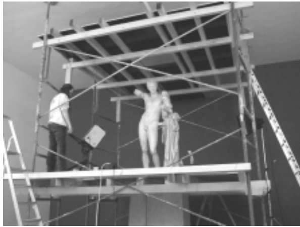
Fig. 1. Scaffolding levels to secure access and stability of laser scanner
